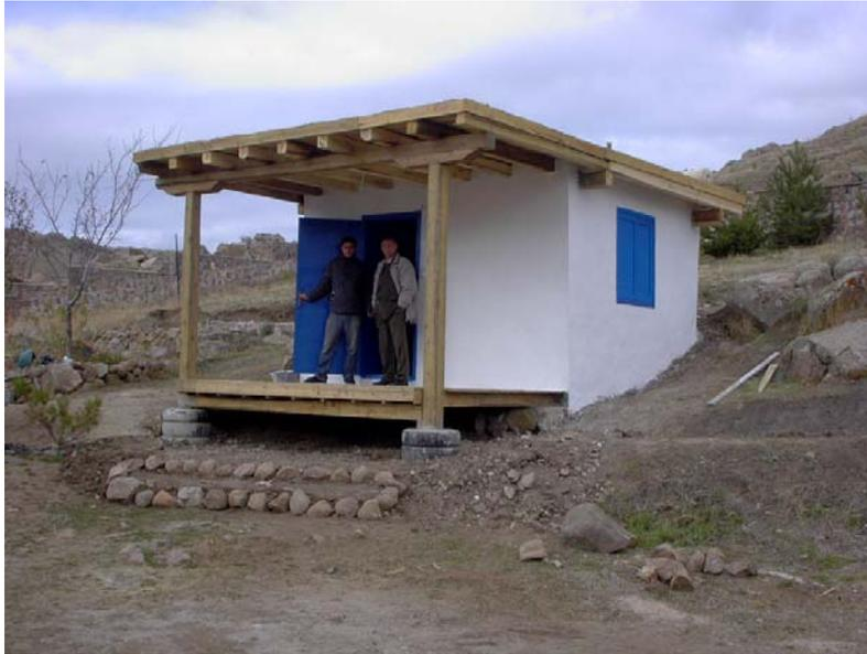
*Figure 14. The mudbrick walls of the unit structure have stone foundations. The flat mud roof, with its timber ceiling and rafters, is supported by beams and posts built into the walls so as to make the structure earthquake resistant.*
