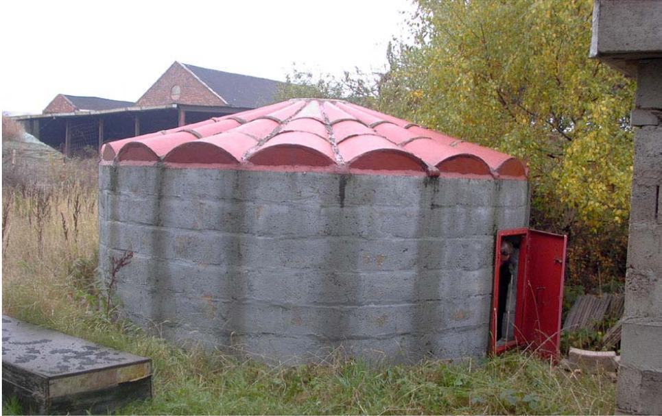
*Figure 11. Cylindrical water tank built from curved interlocking concrete blocks could help solving the seasonal water shortages that occur in many Turkish villages.*
